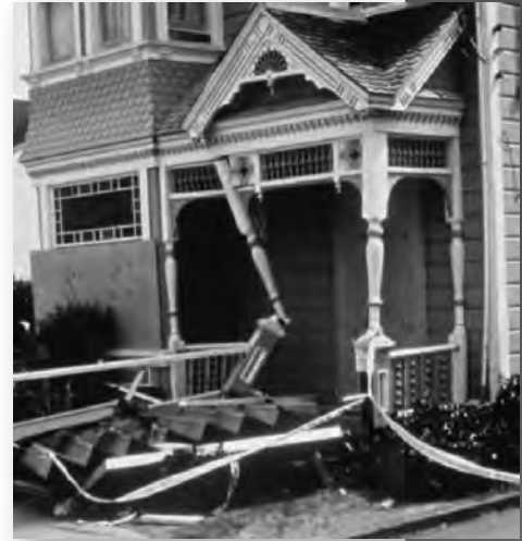
This older home collapsed after earthquake shaking its crawl space (cripple) walls.
