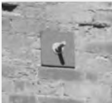
A steel plate with anchor bolts.
