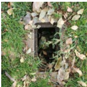
Common Water Meter
